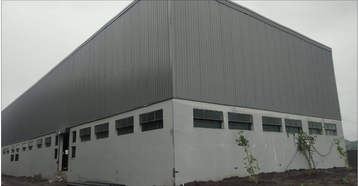
Factory Side View
